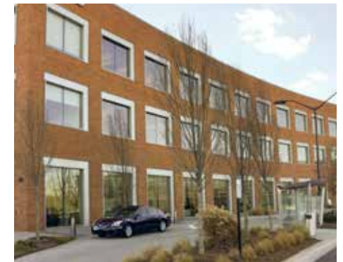
UNC HEALTHCARE HILLSBOROUGH CAMPUS 130,000 SF Physician Center and 68-bed acute and intensive care facility which features medical office, an emergency department, outpatient surgery, as well as a broad range of inpatient services.
