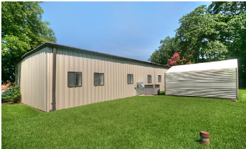
Rear Exterior with Storage Shed
