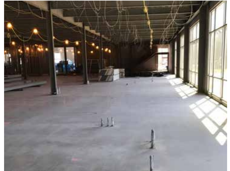
▼ 1ST FLOOR - FUTURE OFFICE AREA
