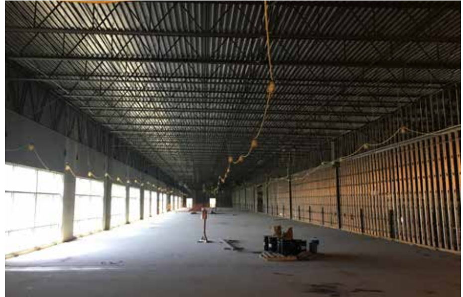
2ND FLOOR - 25,000 SF STRUCTURAL MEZZANINE
