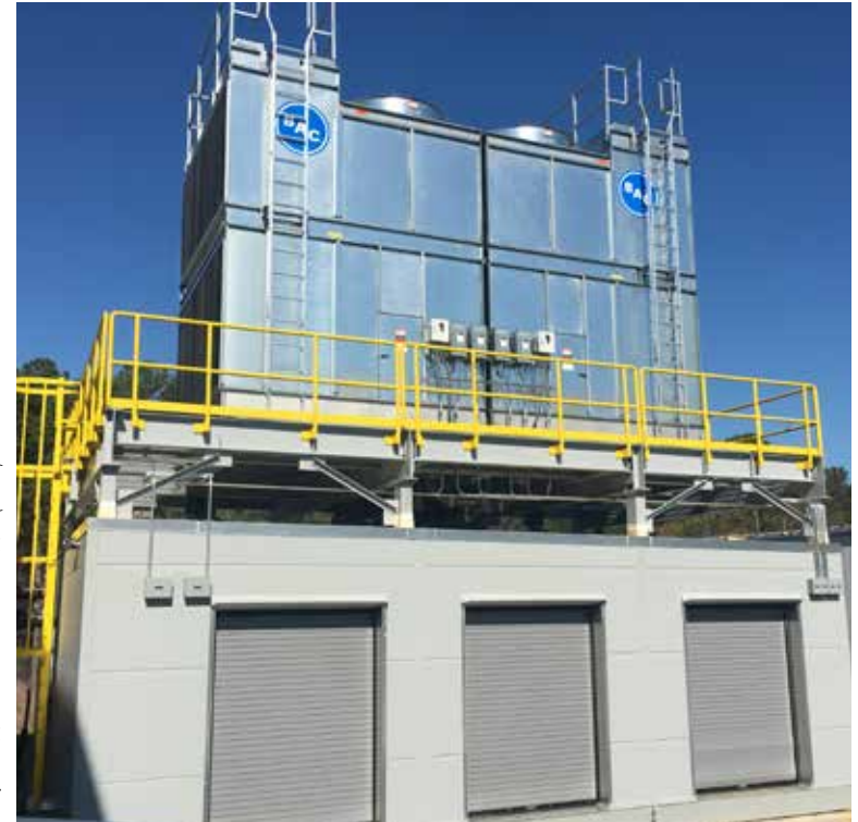
✓ CENTRAL UTILITY BUILDING (CUB)
