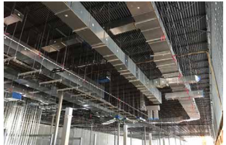
▼ HVAC DUCT WORK PHASE 1 | MANUFACTURING
