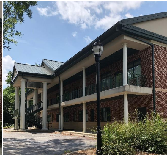
Double Stairwell Access to Second
