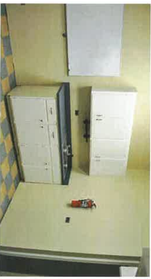
1 ST FLOOR / OFFICE AND BREAK AREA
