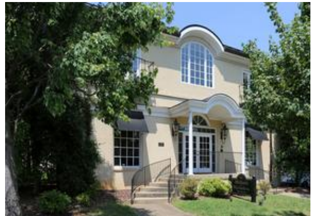
The 107 Glenwood Ave. office building was sold for $1.8 million in April 2016.
